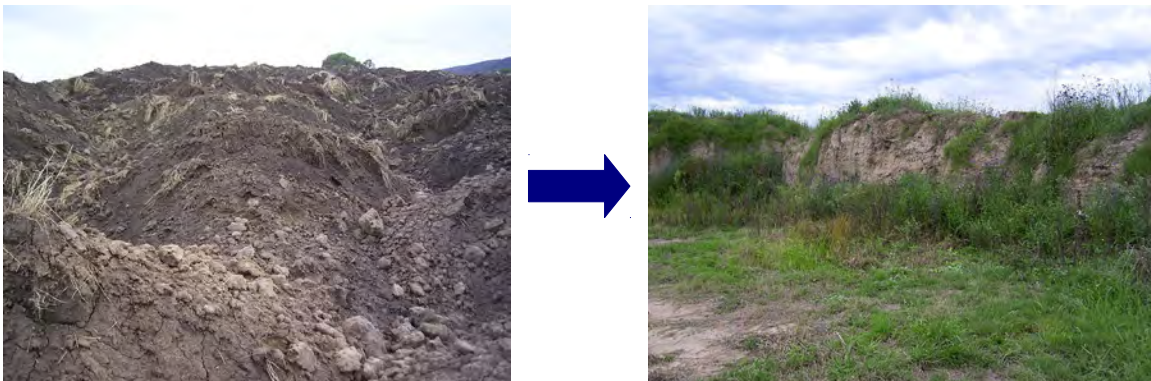
FIGURE 10. Topsoil stockpiles must be stabilized to avoid subsequent mass soil erosion and de-differentiation issues. A fresh topsoil stockpile (left) and an unstabilized stockpile (right) are shown.
